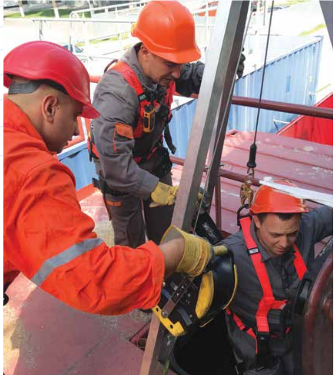
Work Permit, Enclosed Space Entry & Rescue at KMSTC, Ukraine
