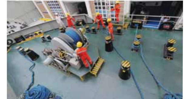
New mooring station at UMTC, Manila
